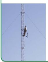
A wind generator tower is very often more expensive than the turbine. The tower puts the turbine up in the "fuel" the smooth strong winds that give the most energy. Wind turbines should be sited at least 30 feet (9 m) higher than anything within 500 feet (152 m).
