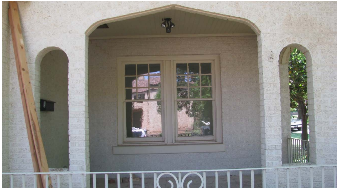
Windows to be removed and replaced with French doors
