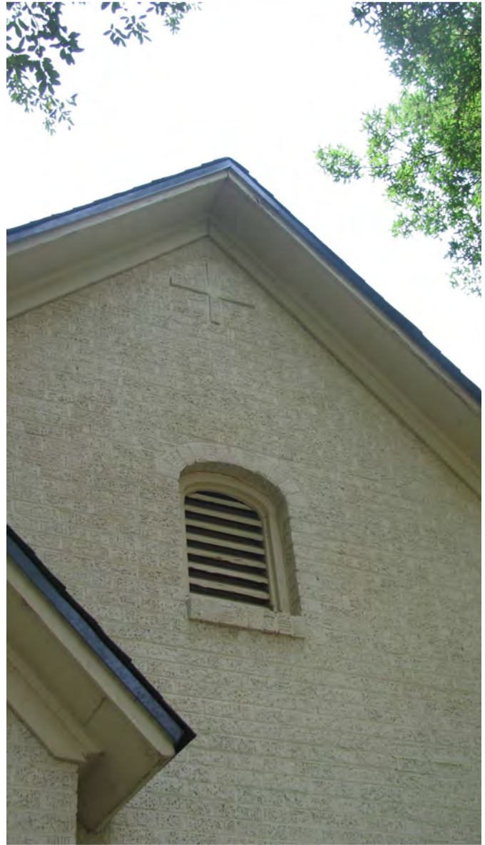
Wood elements of the attic vents and the relief crosses to be painted black. The roof fascia and soffit will also be painted black along the entire roofline.
