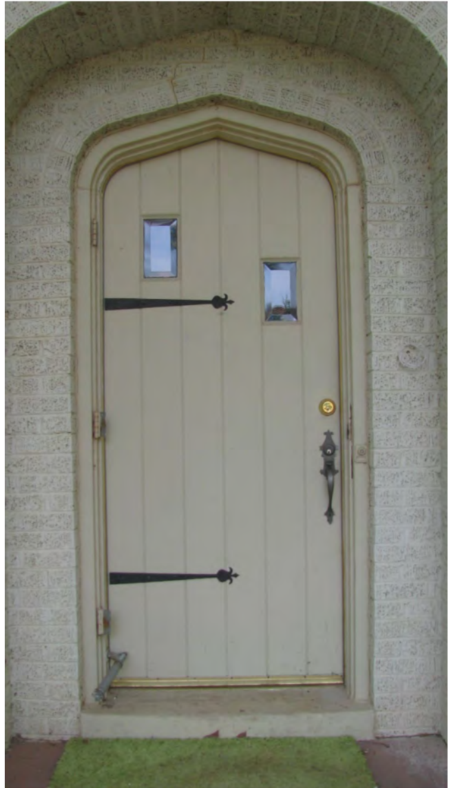
The front door and door frame will be stained.
