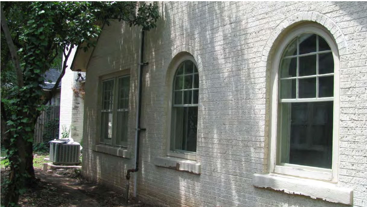
The wood elements of all windows will be painted black. The ledges underneath the windows will also be painted black.
