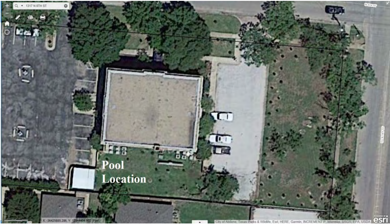
Aerial image showing location of pool
