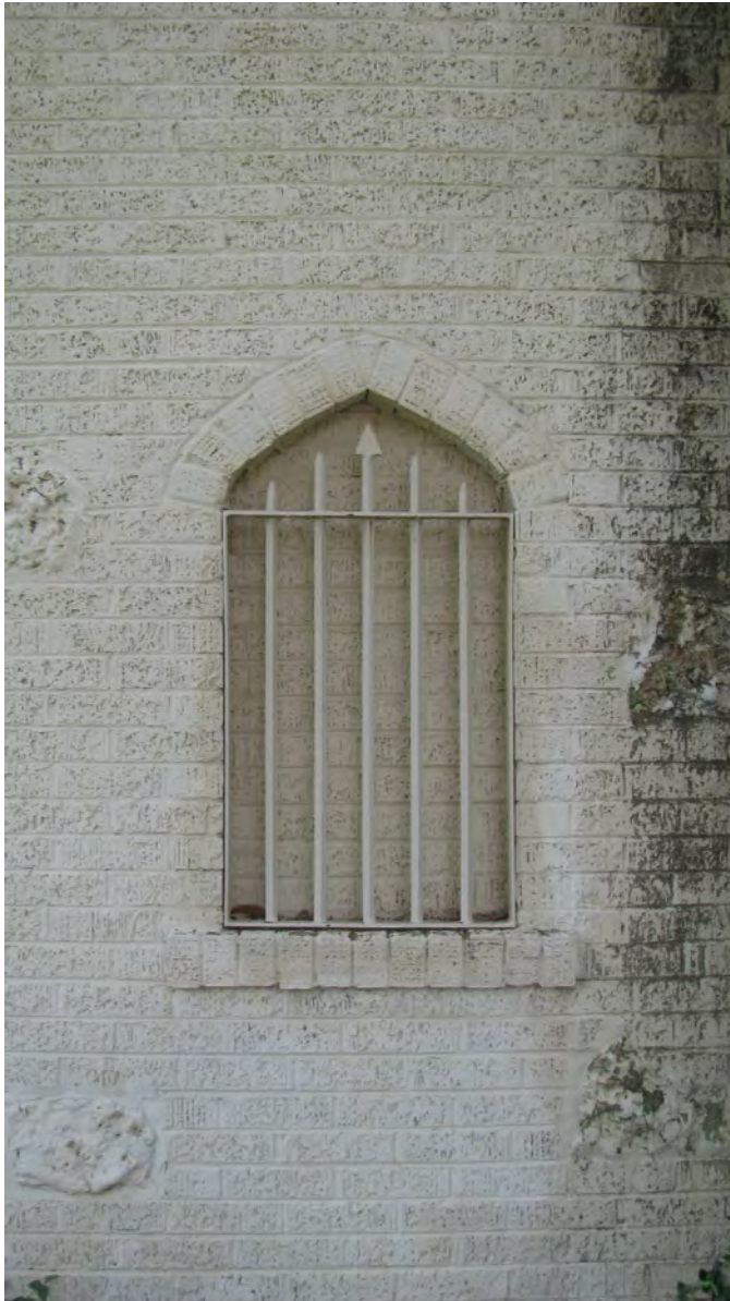
Metal feature to the left of the front door to be painted black. The bricks forming the arch will also be painted black. Bricks forming arches on other front elevation features – front door, porch opening, window – will also be painted black.
